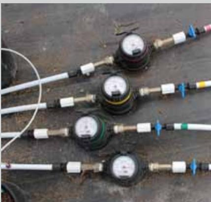
Water meters measuring the volume of water used.
